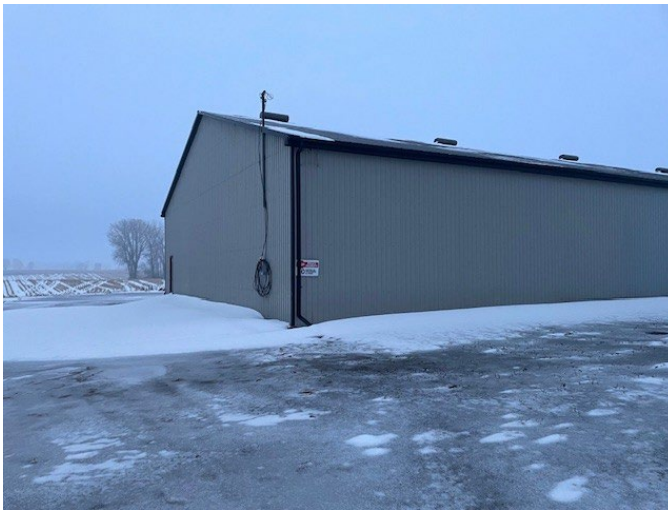
Front facing (south-west) view of structure at 75 Highway 53.
