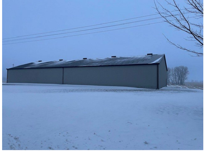
Front facing (south-east) view of structure at 75 Highway 53.
