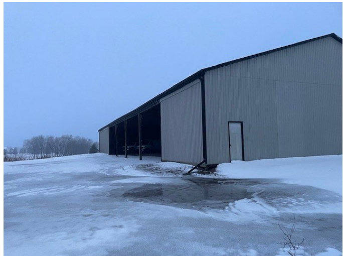
Facing the other side of the structure.
