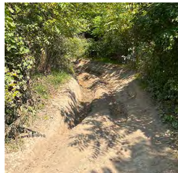
Image 8. Rutting of the trails from motorized vehicles.
