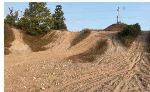
Image 17. Erosion of natural banks caused by motorized vehicles.
