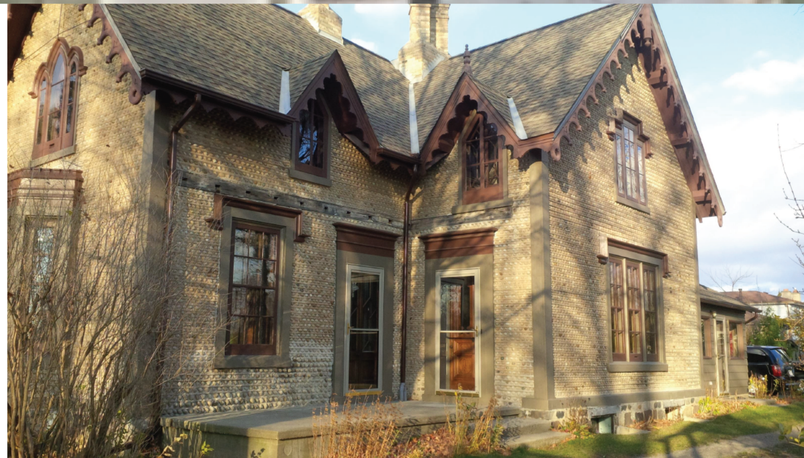
PHOTOGRAPH OF EXISTING CONDITION
