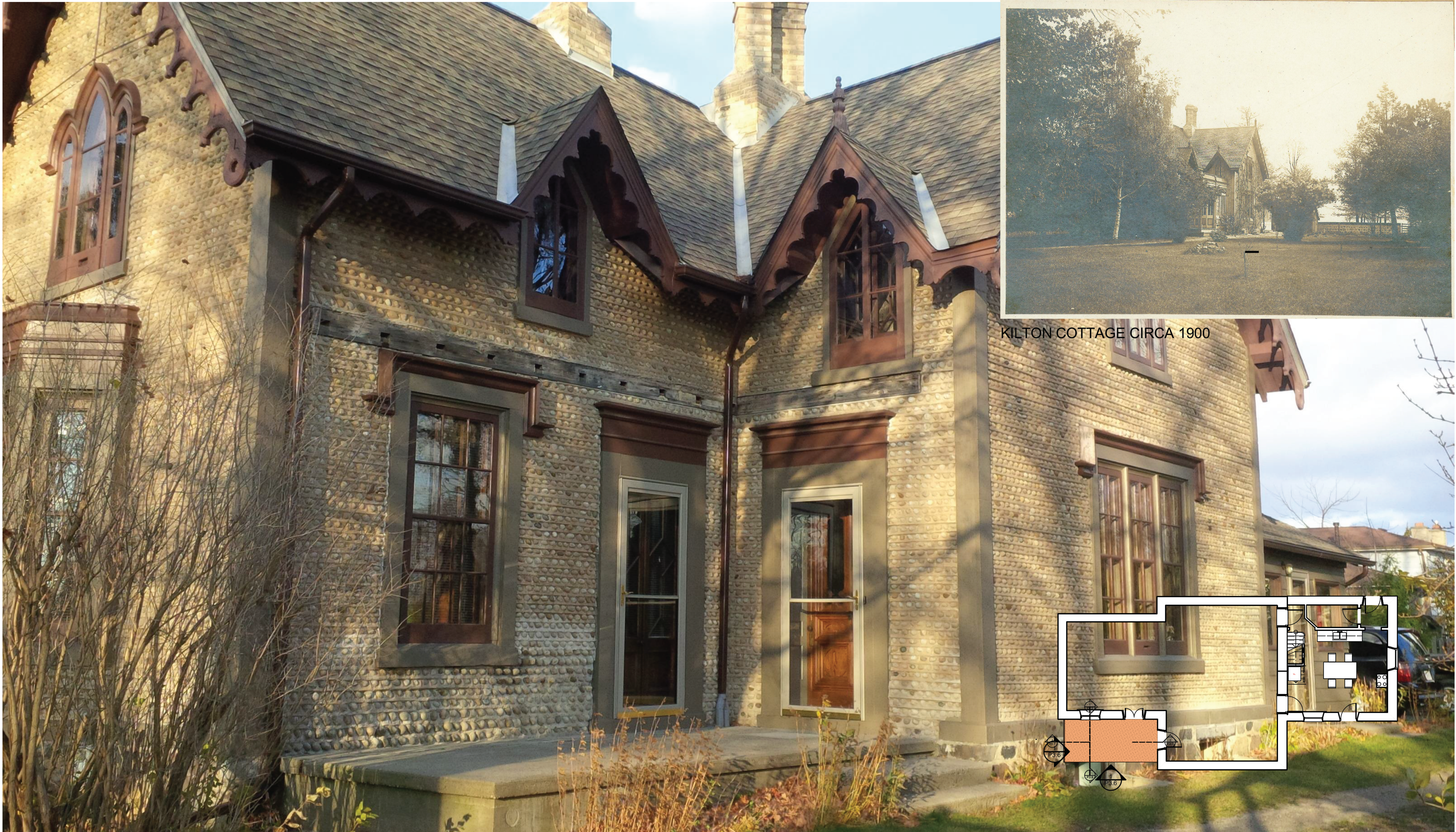
PHOTOGRAPH OF EXISTING CONDITION
