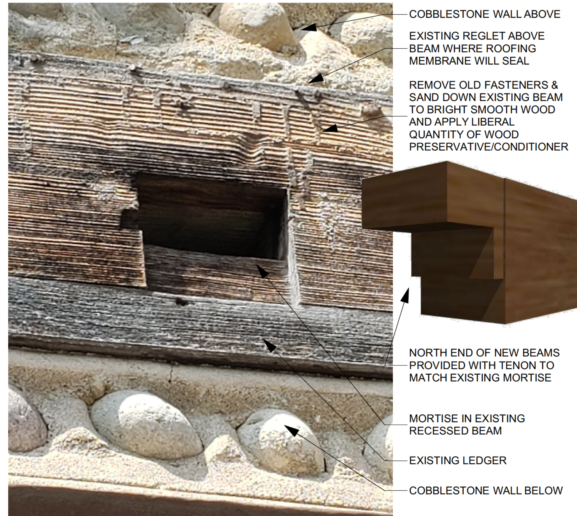
3 MORTISE IN RECESSED BEAM & NORTH END OF JOIST P3.2.7
