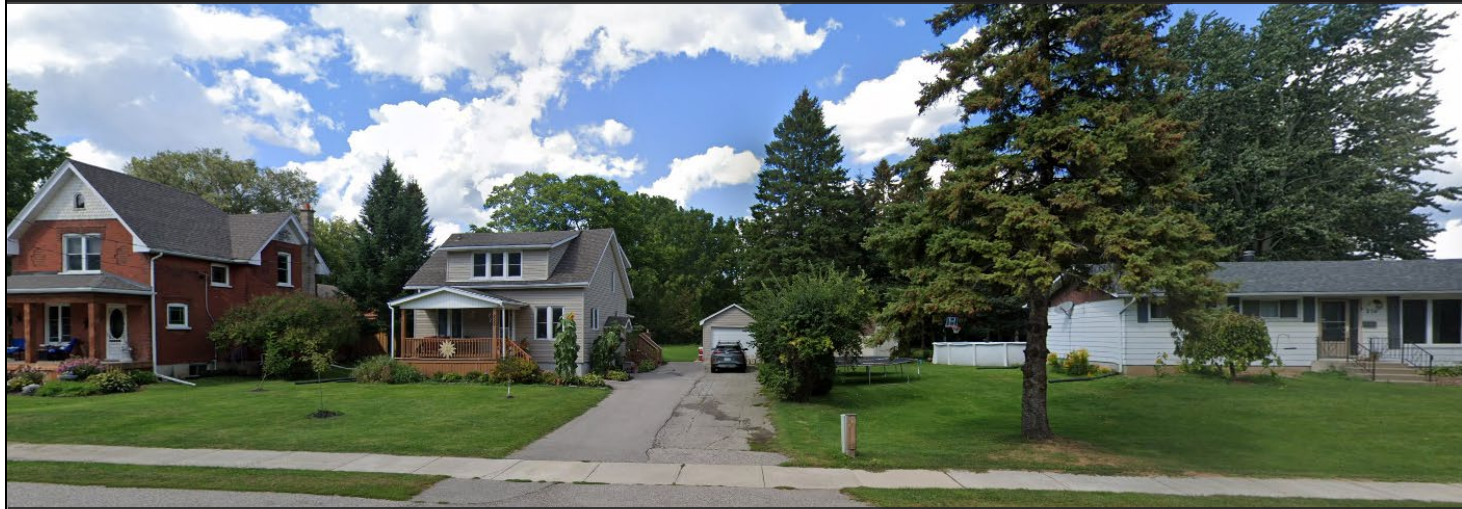
Adjacent Residential Lots (250, 252 & 254 Oakland Road)
