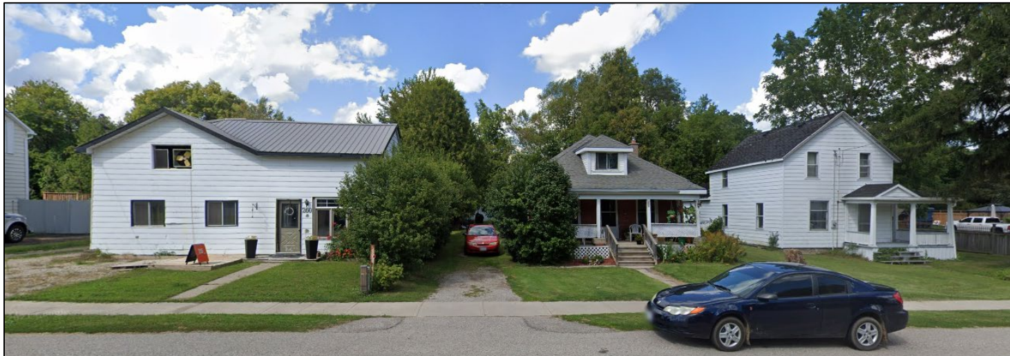
Adjacent Residential Lots (256, 258 & 260 Oakland Road)
