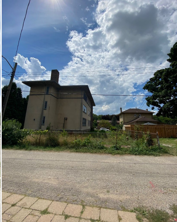
Rear of Existing Building
