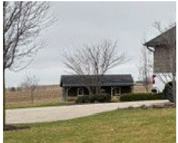
Picture of existing shed.
