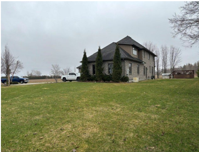
Front-facing (southwest) view from right side of the property.
