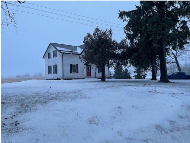
Front facing (south-west) view of 75 Highway 53 property at entrance.
