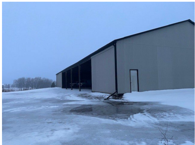
Facing the other side of the structure.
