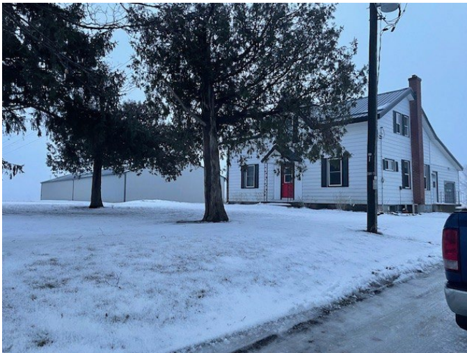
Front facing (south-east) view of 75 Highway 53 property at entrance.
