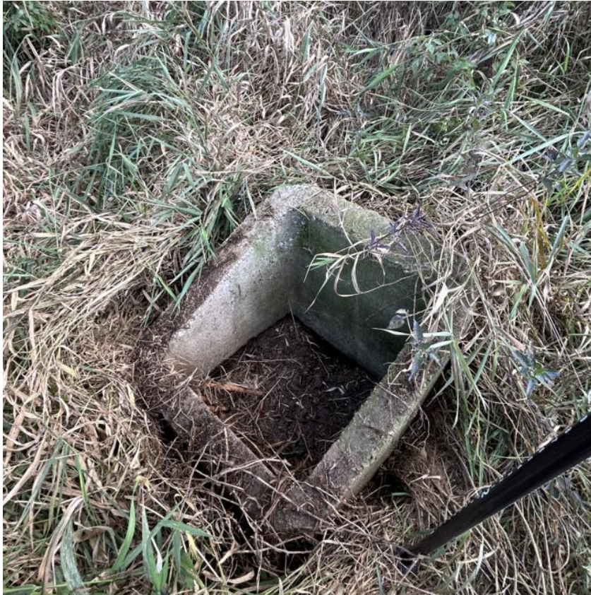
Figure 2 - Existing Concrete Catchbasin Filled with Sediment
