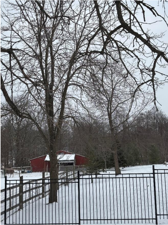
Livestock Barn Located at 76 Hammond Road
